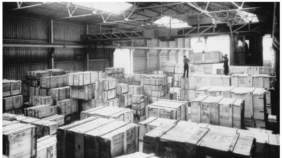
Above, the new warehouse for Howard & Bulloughs' trade at Church. The overhead crane extended over the canal for easy loading.
